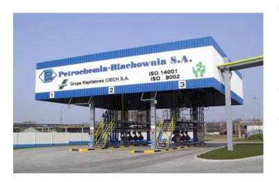
The completely new facility which is located next to the existing tanks ensures tank truck loading by a top loading arm. Vapors from the truck are recovered back into the tank through the vapour arm.
