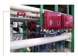
Hydraulic connections are made with elastic hoses using quick couplers which reduces the installation and service costs and eliminates the transmission of mechanical vibrations and shocks.
