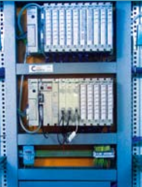
PLC part of automation system.
