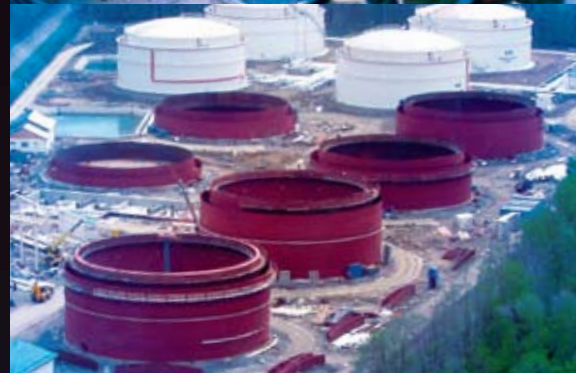
Erection of storage tanks in Sedlnice (CZ).
