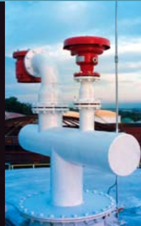
Protego end-of-line flame arresters.
